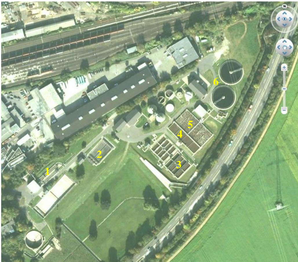
Figure 2-3. Overview of Frechen municipal wastewater treatment plant with (1) grease trap, (2) primary settlement tank, (3) biological phosphorus tank, (4) denitrification tank, (5) nitrification tank and (6) secondary settlement tanks
