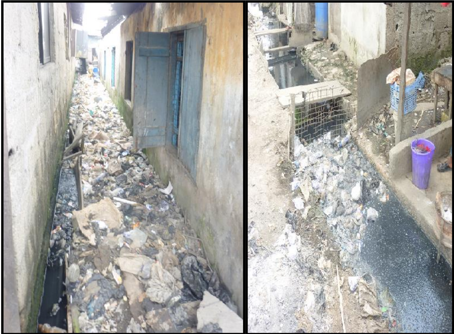
Figure 8: Silt accumulation, man-made blockages, and rubbish build up Source: own photos from the field, 2011
