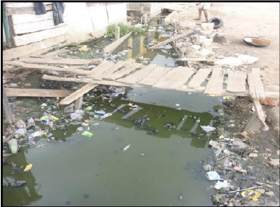
Water logging in the drainages of Badia slum Pictures by Nsorfon, 2011
