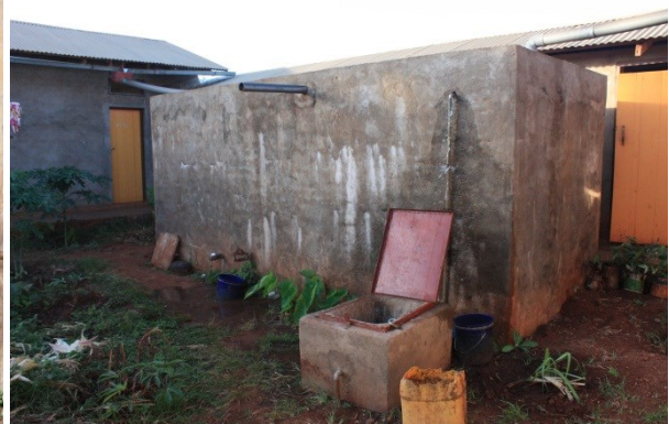
Figure 19. A private water connection with a concrete lined tank in Endamarariiek, 03.01.2010
