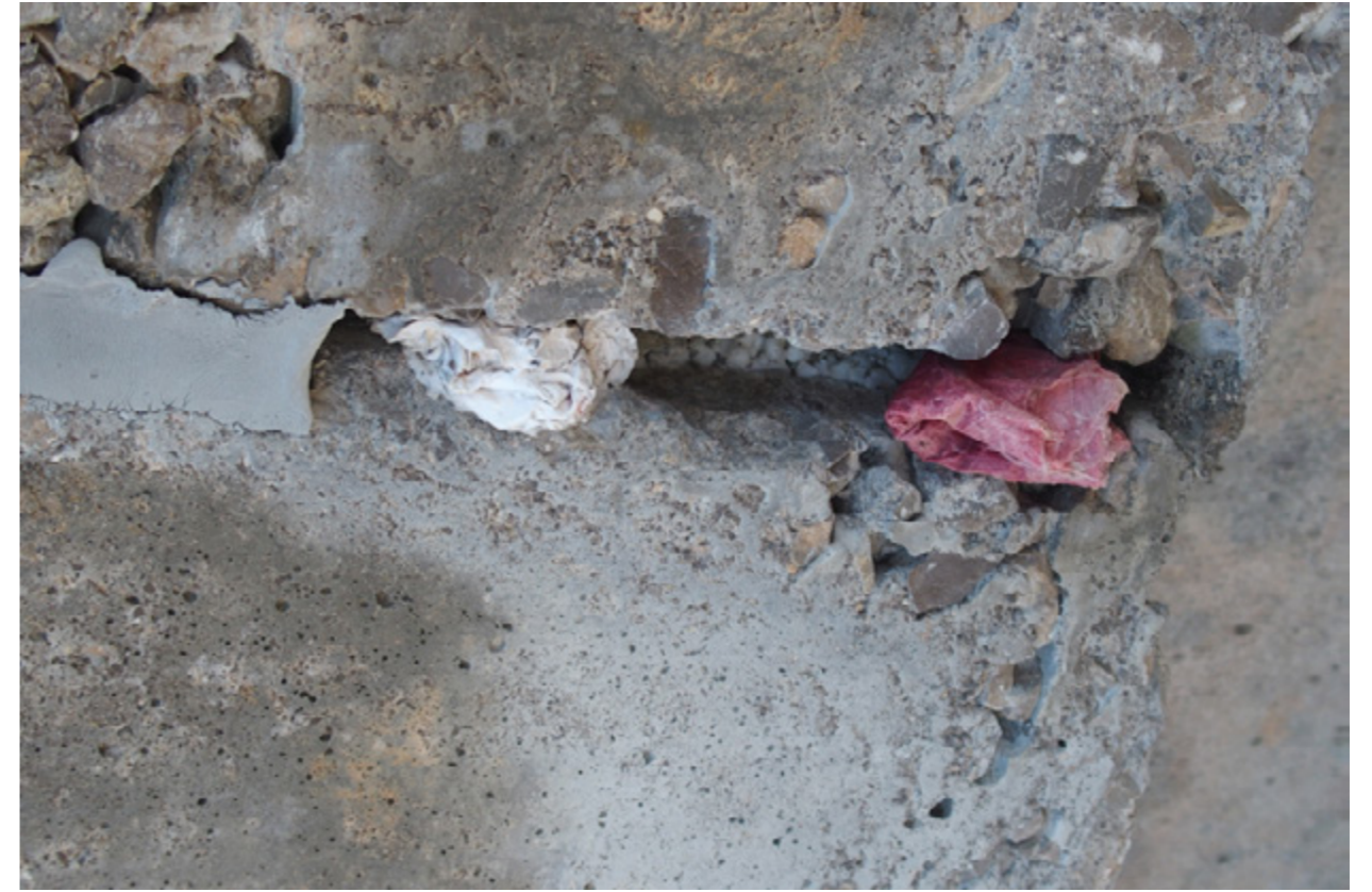
Hidden in the wall (A. Mietzner 2017)
