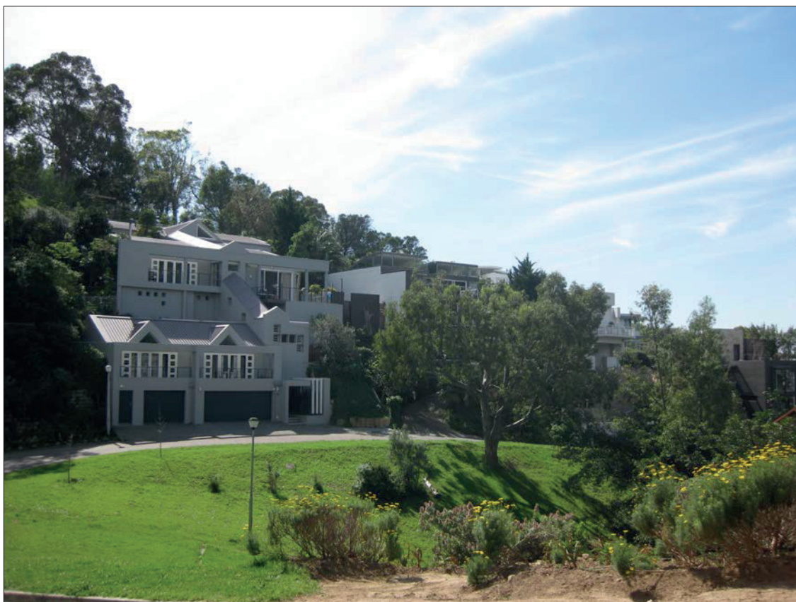
Photograph 4: Modern architecture on Leeukloof Drive, 2015.
