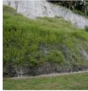
d) Stapled soil retaining structure with green cladding.
