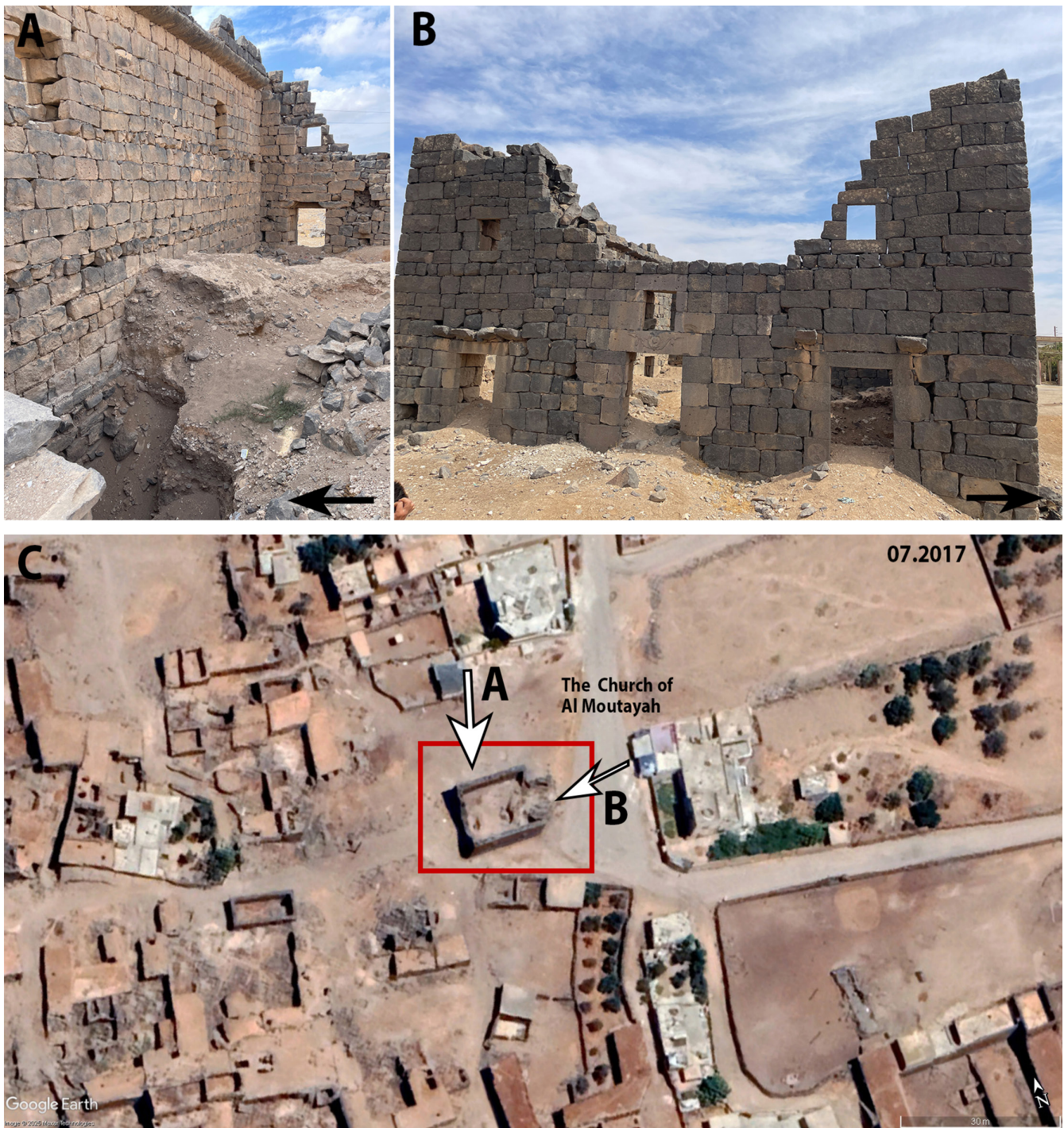
FIGURE 6 | (A and B) Looting pits documented in the church of Al Moutayah, extending beyond 2 m in depth, increase the likelihood of the wall collapsing in the future. The severity of this damage cannot be accurately assessed using satellite imagery alone, highlighting a key limitation of this method. (C) The church of Al Moutayah on satellite imagery in 07.2017 (Image 2025 Maxar Technologies. Used in accordance with the Google Maps/Earth terms of service for research purposes).
