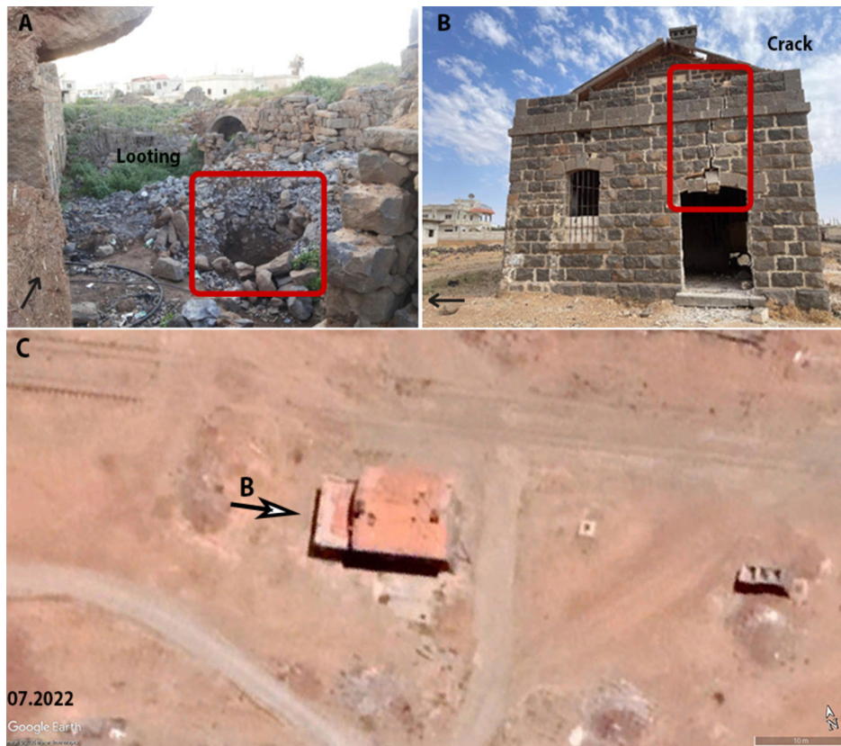
FIGURE 5 | (A) Evidence of explosive use in looting at the ancient town of Saida Village, documented during a 2015 field visit (Al Kassem 2016). This mechanism of looting was not detected using satellite imagery, and only visible in field visits. (B) Cracks in the walls, looting of the doors and ceilings, and felling of the trees in the periphery of the Al Teibeh station. Again, none of these damages were clearly visible in satellite imagery, as can be seen in the train station of Al Teibeh in (C) (Image 2025 Maxar Technologies. Used in accordance with the Google Maps/Earth terms of service for research purposes).
