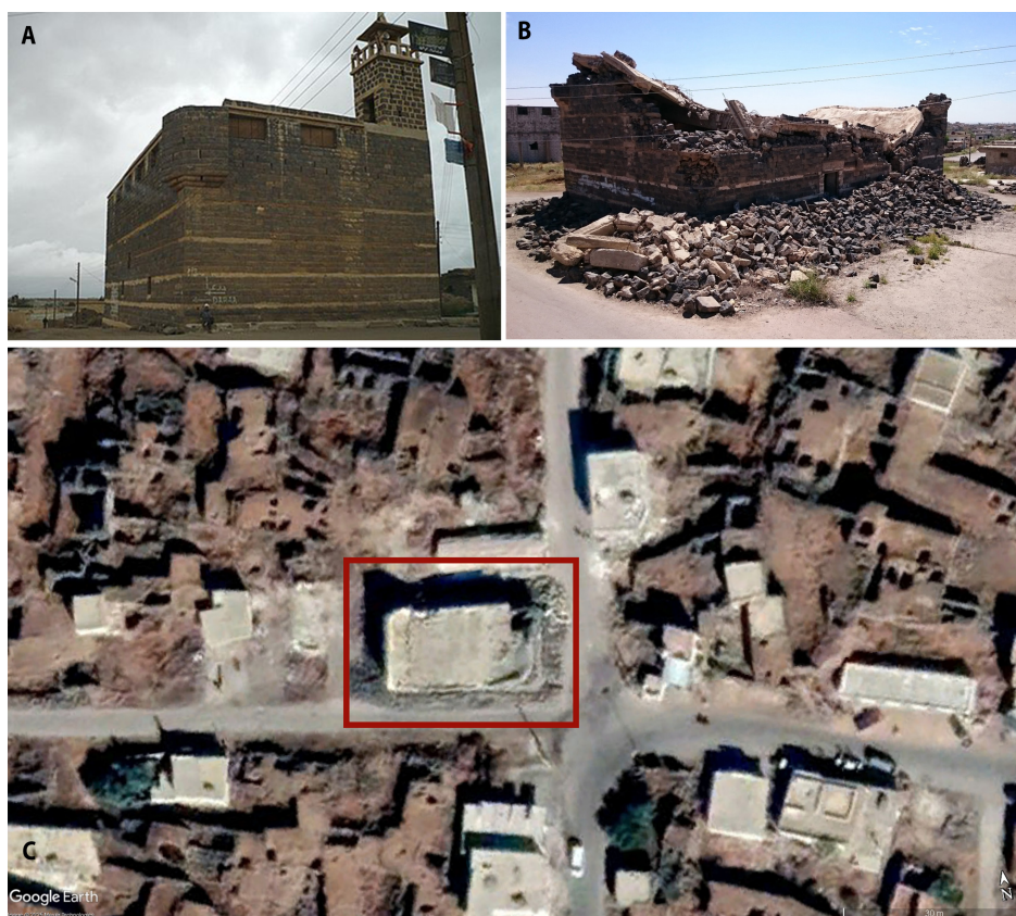
FIGURE 13 | (A) Al Omary Mosque in Ma'araba before sustaining damage, originally consisting of two floors. (B) The mosque after experiencing structural collapse during armed clashes in 2014, as documented during field visit in 2015. (C) Satellite imagery taken in 2019 shows the location of the mosque (Image 2025 Maxar Technologies. Used in accordance with the Google Maps/Earth terms of service for research purposes). This type of architectural deterioration is challenging to detect using satellite imagery alone, emphasizing the importance of ground-based assessments.
