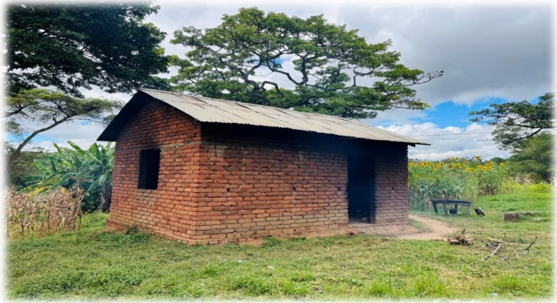
Figure 11: Communal kitchen at Kidugala in Waging'ombe District, Njombe region 341
