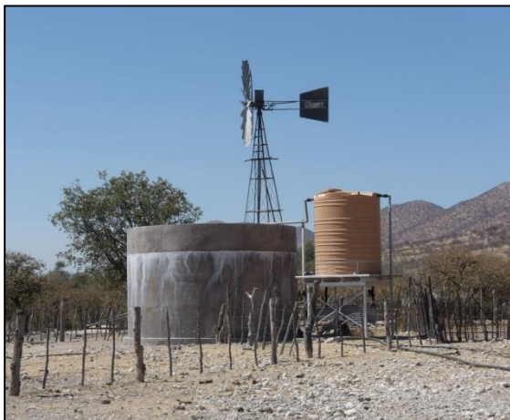
Image 17: Wind pump and reservoir, /'Aub Pos, Kunene South
