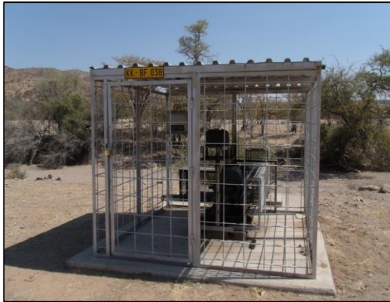
Image 14: Diesel pump installation, Renosterkop, Kunene South
