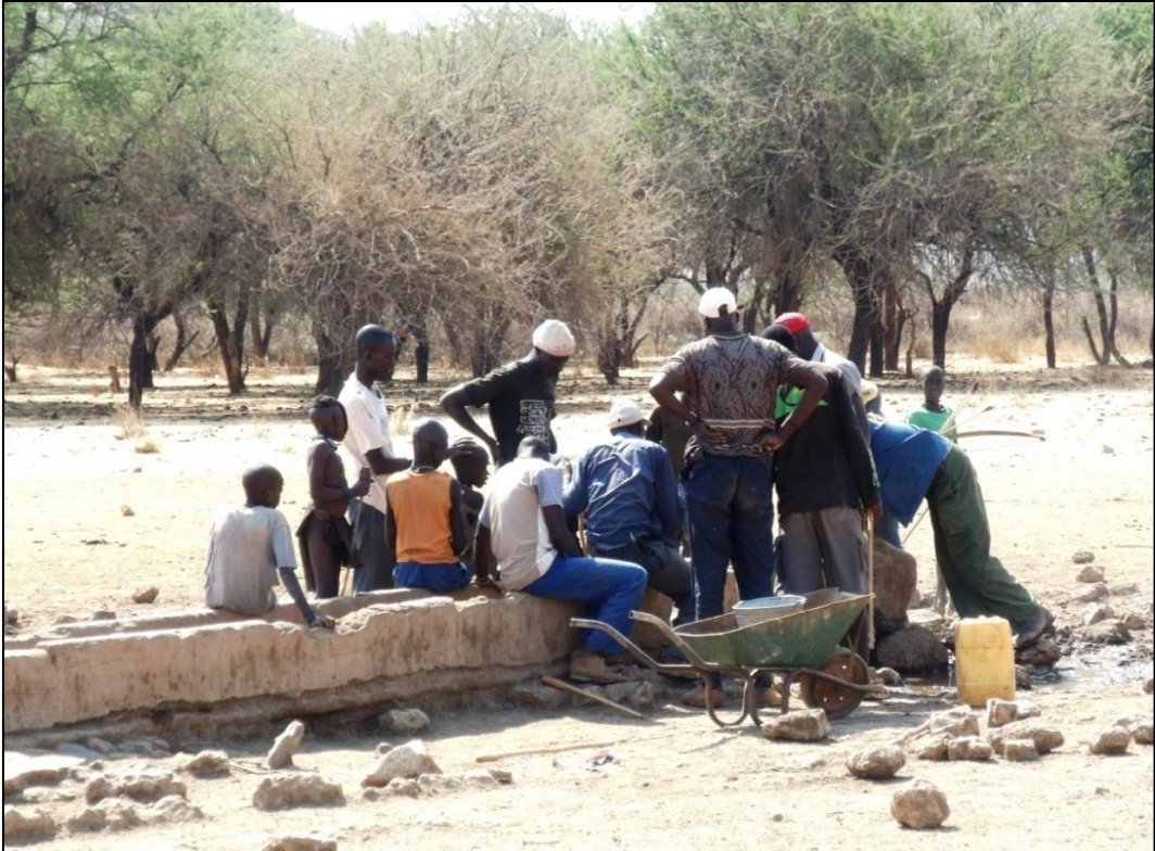
Image 11: - Communal repairs to the water reservoir in Ondjete, Kunene North
