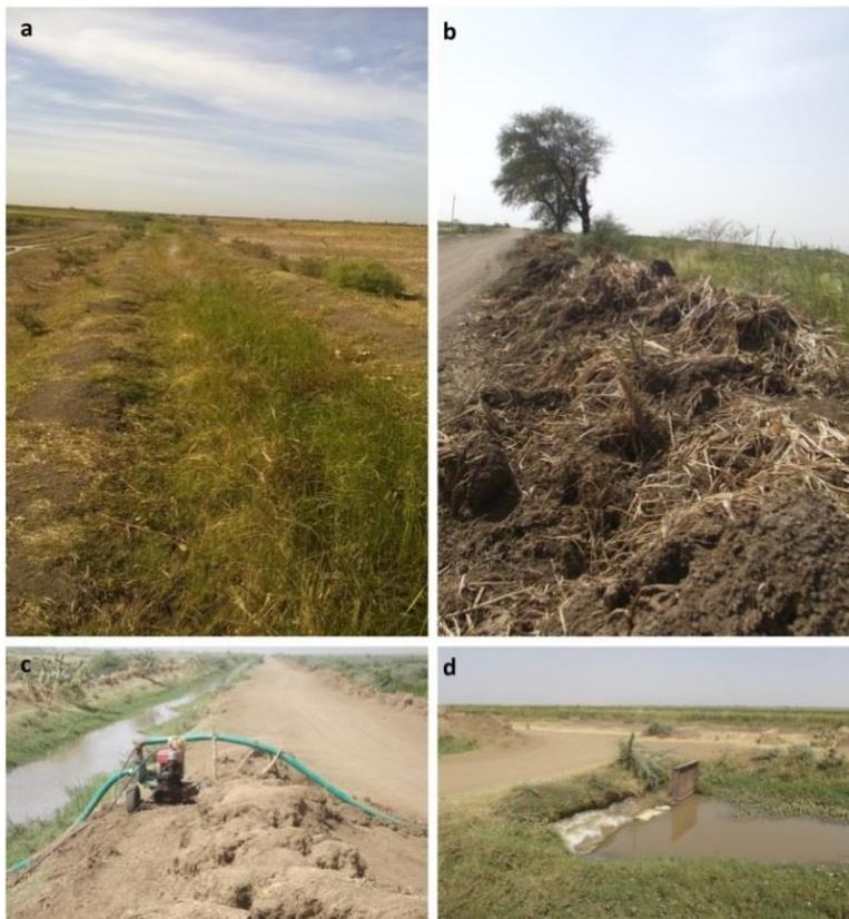
**Fig. S5.2.** Problems in the irrigation canals in the Gezira Scheme: (a) weeds, (b) siltation, (c) improper maintenance resulted in different levels in the canals and (d) broken water gates.
