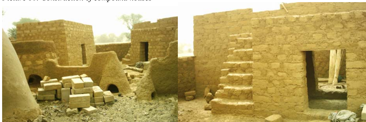
Picture 10: Construction of compound houses
