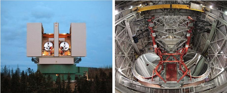
**Figure 1.6:** *The Large Binocular Telescope in September 2007: The two primary mirrors and prime focus cameras are installed. The other mirrors and some swing arms are still missing. (image credit: David Harvey)*
