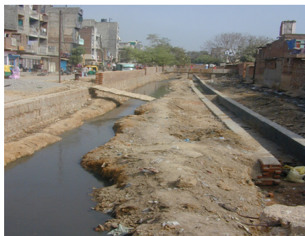
Open Drain (S2) own photo
