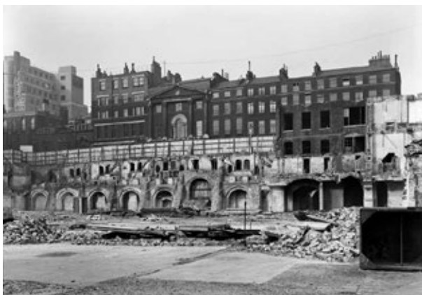
8 The remains of the demolished Adelphi Terrace in 1936
