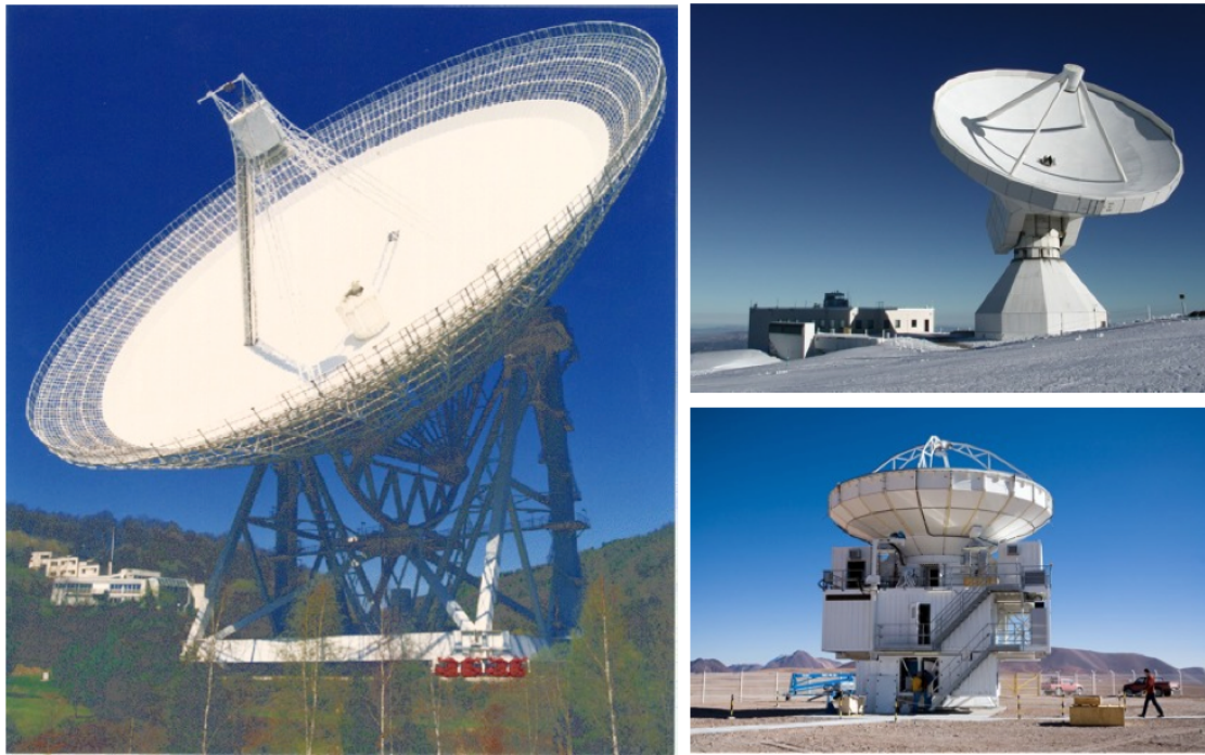
Figure 4.3: The radio telescopes used in the F-GAMMA project. Left: the Effelsberg 100 m telescope; upper-right: the IRAM 30 m telescope; bottom-right: the APEX 12 m telescope.
