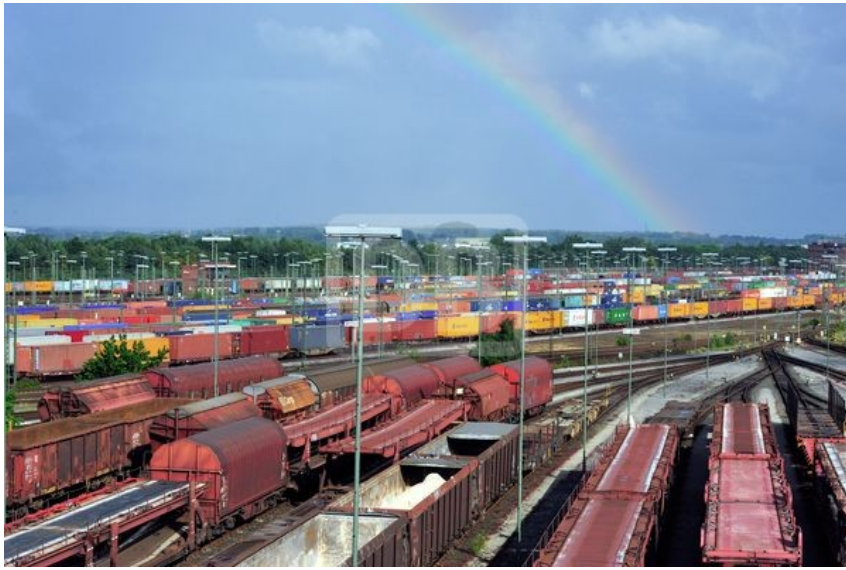
Figure 3: Maschen, shunting yard (DB13244) by Volker Emersleben. Loaded and empty freight cars are assembled to trains together in shunting facilities often equipped with (limited) operational storage. Picture taken from https://mediathek.deutschebahn.com by courtesy of Deutsche Bahn AG.
