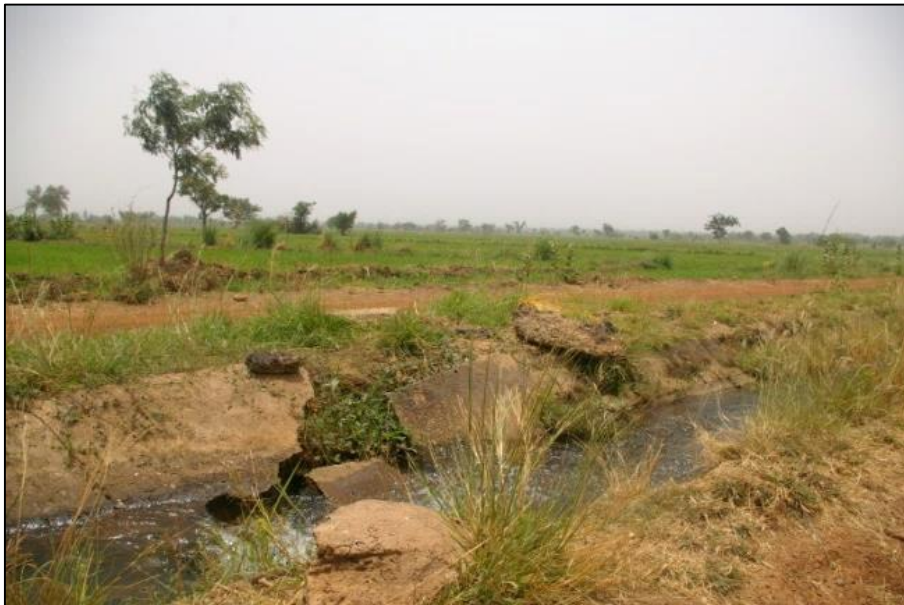
Photo 9: Broken sublateral canal serving low lands near Bui (own photo, 2011).
