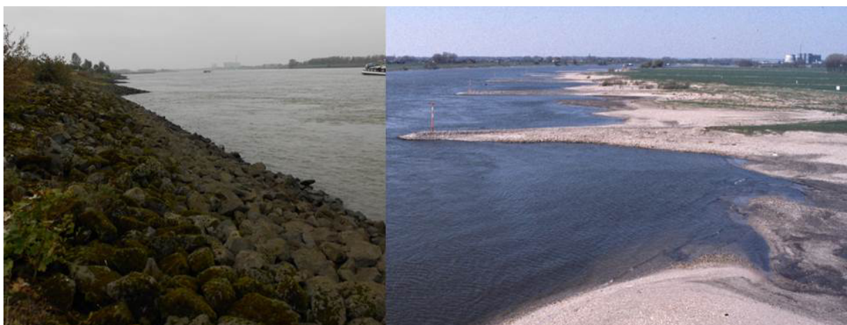
Figure 4. Artificial banks at the Lower Rhine: exclusively riprap (left, photo: S. Gertzen), and large groin fields (right, photo: J. Borchering).
