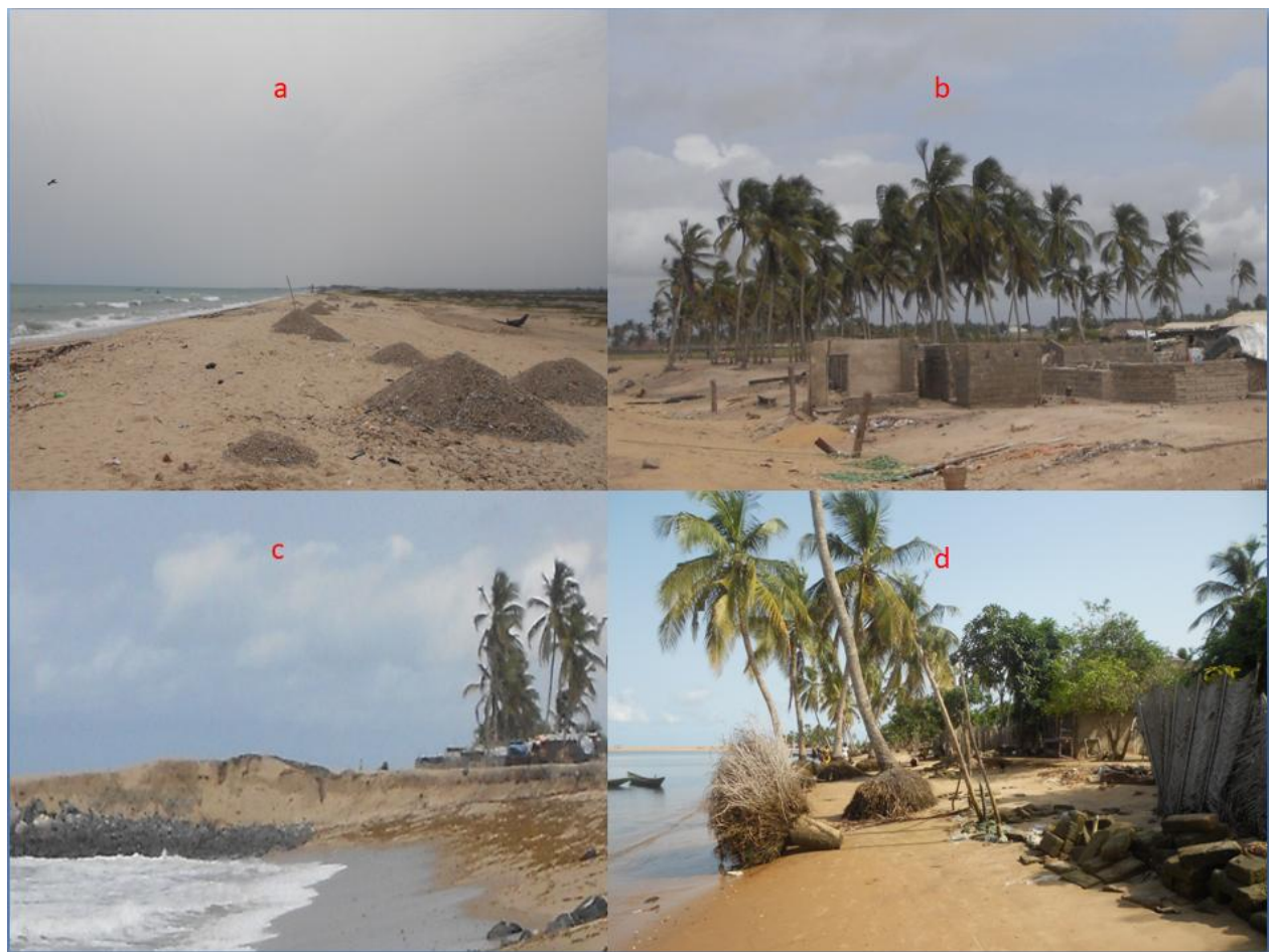
Fig. 5: All the above pictures were taken during my fieldwork in 2019. Picture ‘a’ shows the harvesting of coastline stones for construction purposes along the coastline of Akplabanya in Ada-West, picture ‘b’ shows the abandoning of a structure along the coastline of Otopke in Ada-East due to the impact of coastal flooding, picture ‘c’ shows renewed erosion on reclaimed land (a part of the sea defense project) along the coastline of Otopey-Ada, and picture ‘d’ shows the gradual erosion of coconut trees along the coastline of Azizakpe-Ada.
