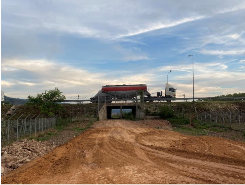
Figure 22. The culvert of Thai Lao Friendship Bridge No.4. Photographed June 11, 2020
