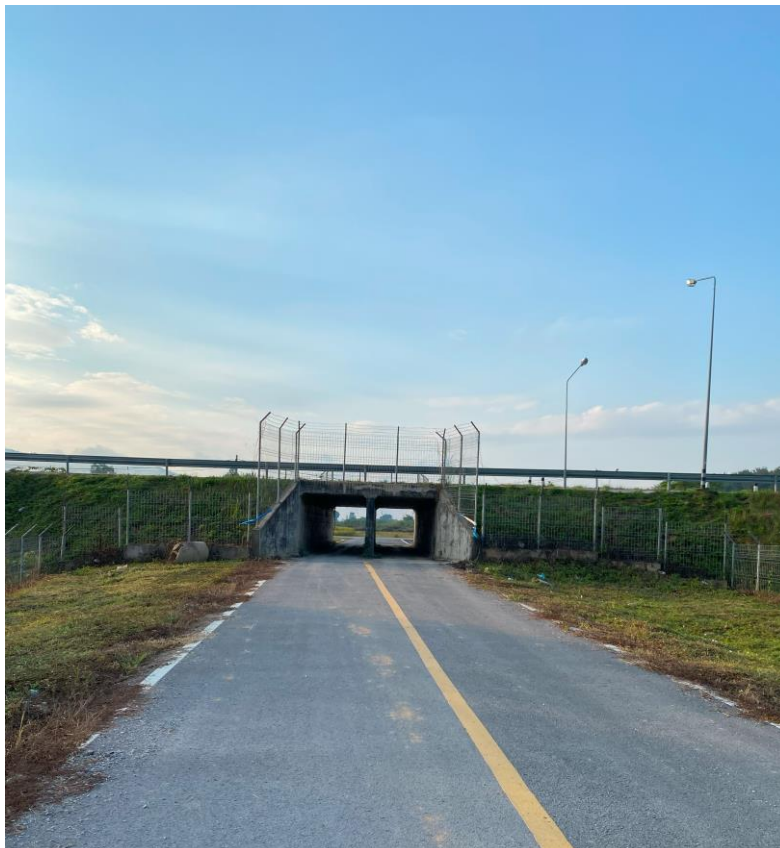
Figure 23. The culvert of Thai Lao Friendship Bride No.4. Photographed December 12, 2021
