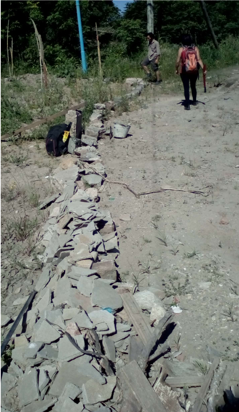
Figure 27: The “trench”. Photo by Vanina Santy. 2018.
