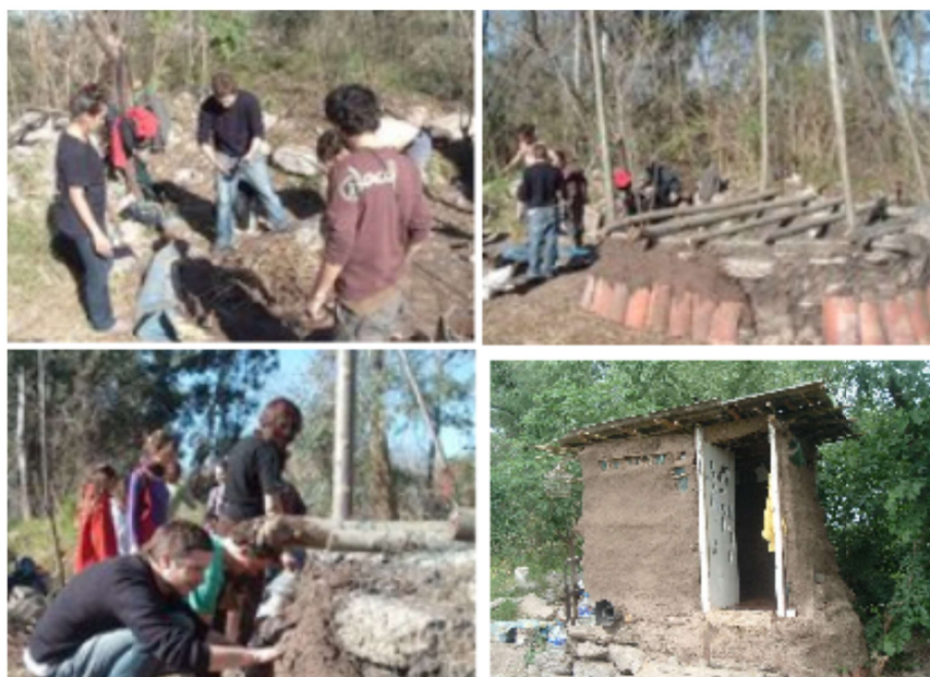
Figure 21: Collective construction of the dry toilet , with the participation of the assemblies and the neighbourhood’s children. Author: Villa Corina Civil association. August 2011.
