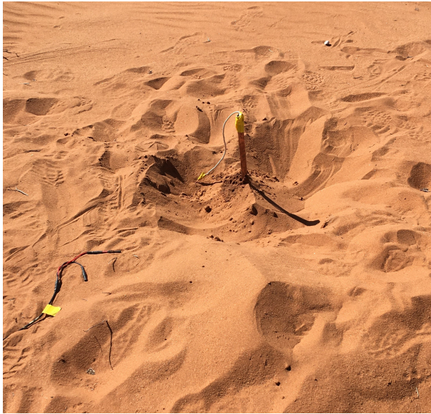
Figure 4.8: Installed copper pipe electrode used for the grounded dipoles for the AMT soundings. The electrodes were approximately 70 cm long and had a diameter of 2 cm. The walls of the pipe were 2 - 3 mm thick.
