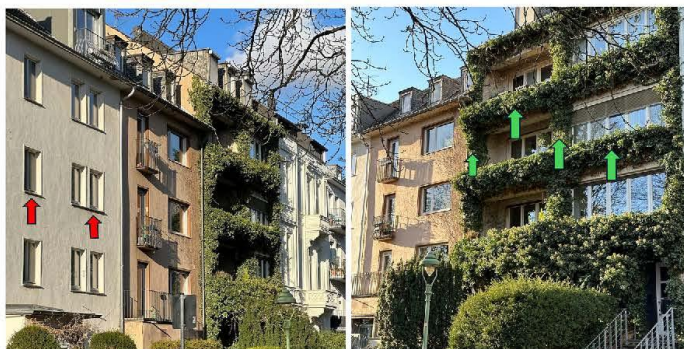
Figure 1: An image of the ground-based façade greening under investigation; with arrows showing locations of data loggers.
