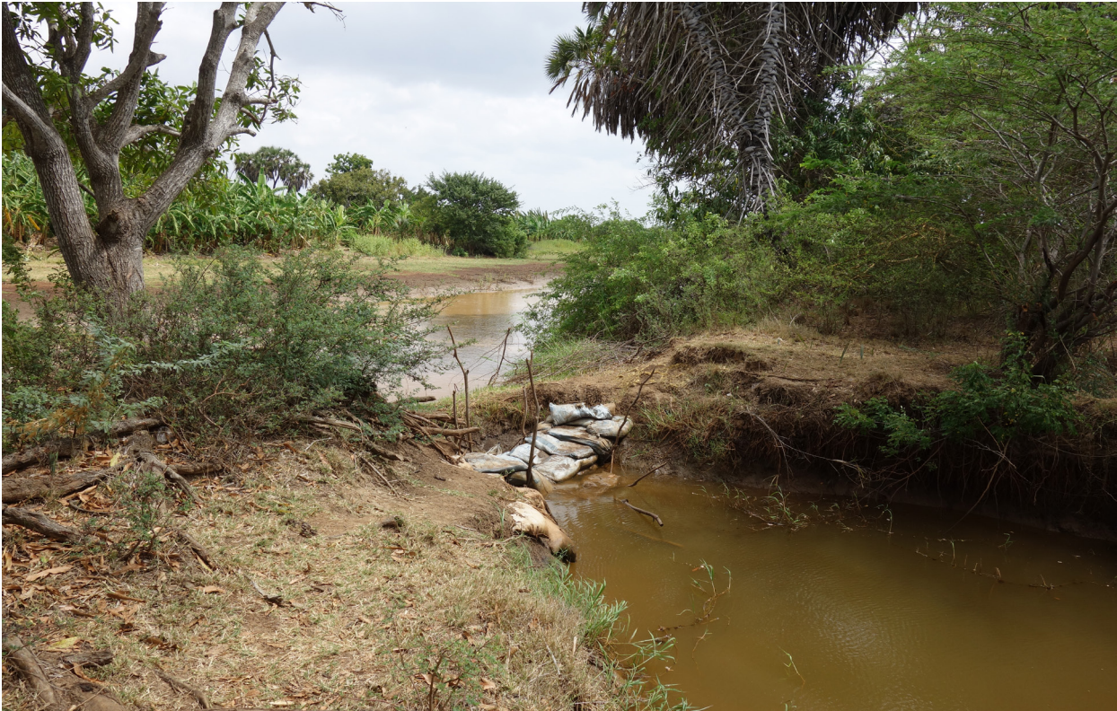
Inland-flowing streams with brackish water threaten to contaminate the main river. In the absence of (governmental) spillover blockages, sandbags and sticks are used to hold back the brackish water.
