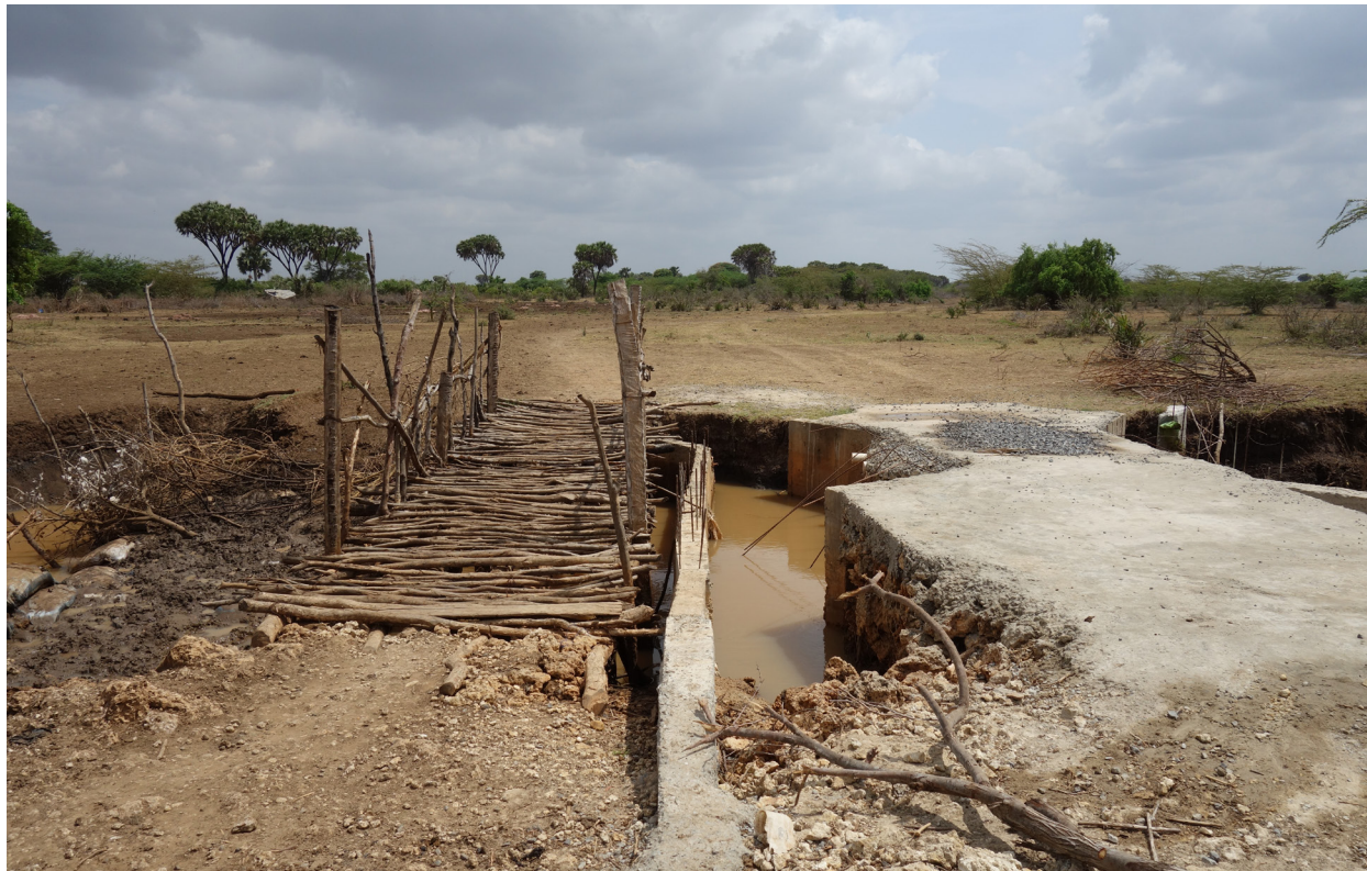
Spillover blockages made out of cement allow the fresh water to flow during the rainy season, while blocking brackish water in the dry season. However, they are rare, might be “left back” after the water found new ways and, in the absence of governmental maintenance, disintegrate. A bridge assembled out of sticks by the local communities allows for light transport and, with its localized malleability, contrasts with the cement blockage.
