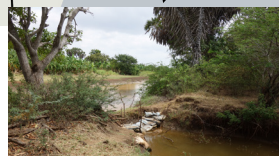
Inland flowing streams with brackish water threaten to contaminate the main river. In the absence of (governmental) spill-over blockages, sandbags and sticks are used to hold back the brackish water.
