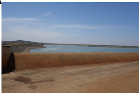
Masinga Dam is one of five dams along the Tana river. Located hundreds of kilometers upstream from the delta, they together generate 70 percent of the country's hydropower. Their construction decreased peak flows, runoff and meandering of the Tana and the related deposition of sediments, which resulted in a reduction of the floodplain fertility and of riverine forest. This again adversely affects deltaic flood recession agriculture, livestock keeping, and fish production.
