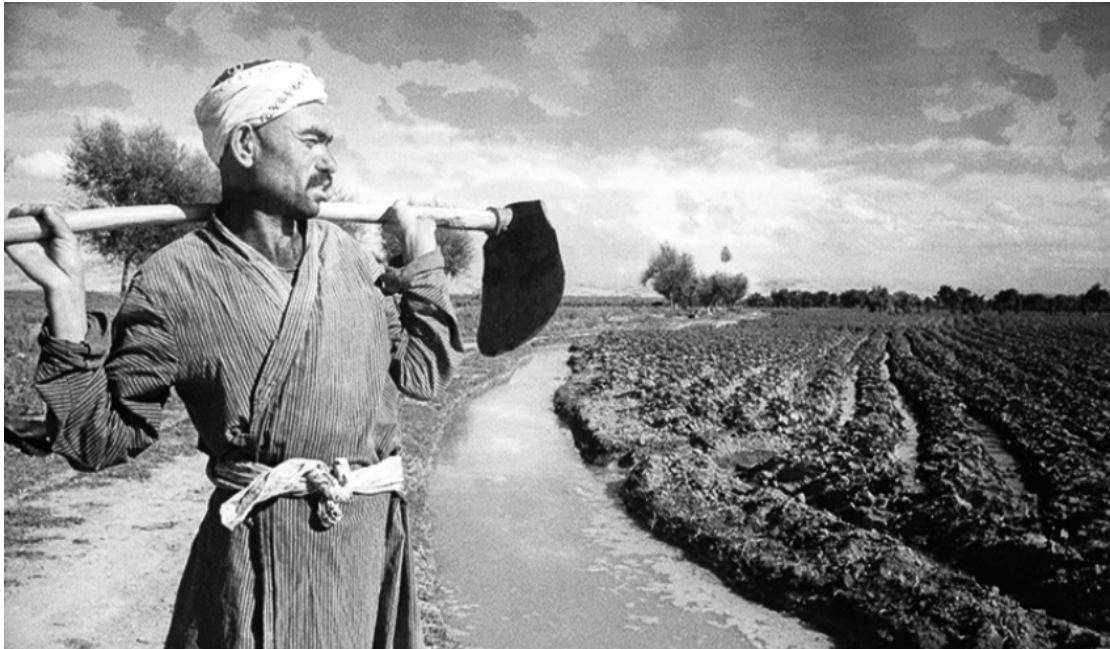
Local water manager carrying out repair work on major canal, Ferghana valley, ca. 1939.
