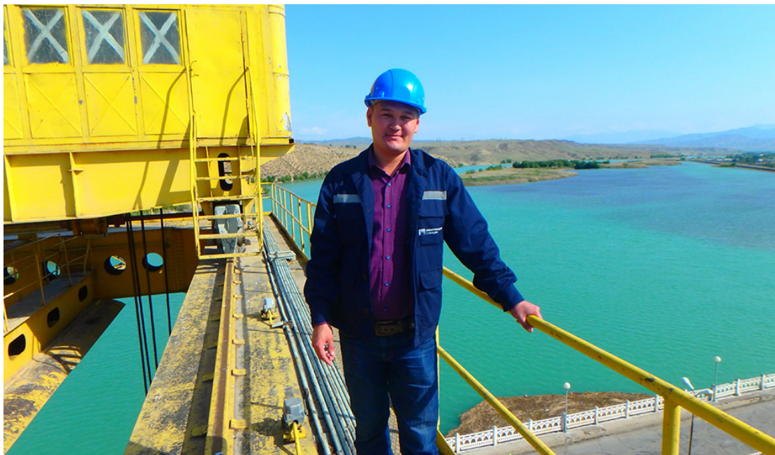
Dam worker on Uch Kurgan Hydropower Station, now militarized as part of the Kyrgyz-Uzbek border.
